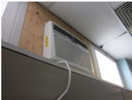
Valleyview Middle School Insulation Opportunity
