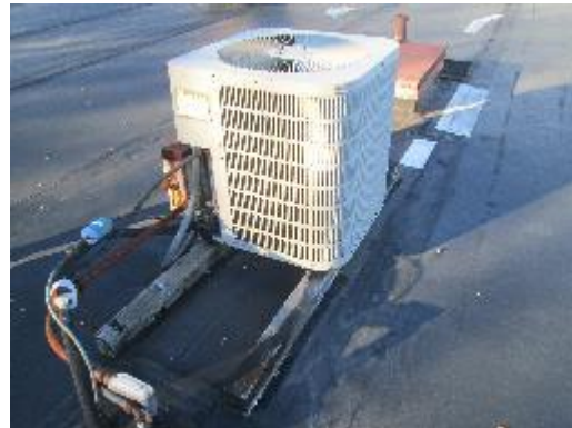
Split system serving IT Closet – Riverview Elementary School and Valleyview MS Guidance
