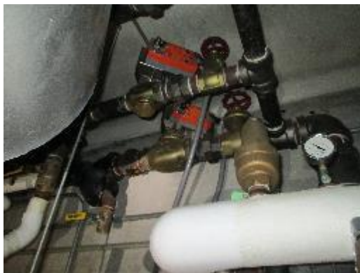
Riverview ES Un-insulated Hot Water and Steam Piping
