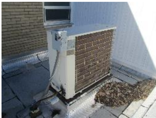
Split system serving IT Closet – Riverview Elementary School and Valleyview MS Guidance
