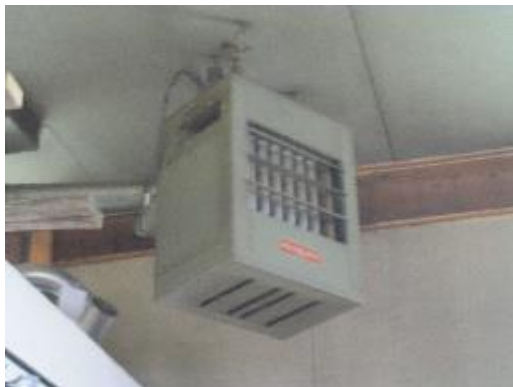
Bus Garage Unit Heater Bay 1
