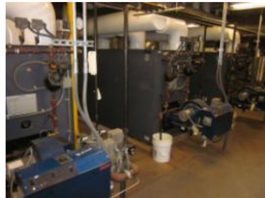
Riverview Elementary School – Boiler Burners
